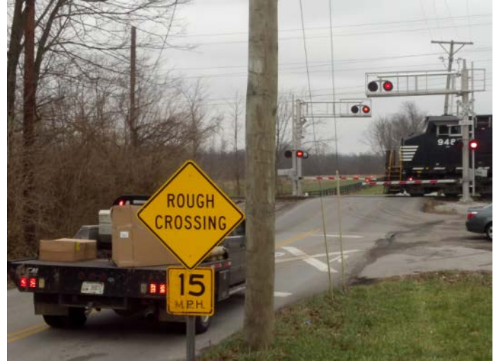
Figure 2. Brannon Rd Crossing
